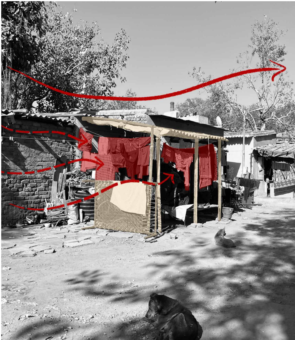
Figure 5.2.5: The image highlights having an extension in front of the houses, which acts as a barrier to prevent wind from entering. The space is usually covered with clothes to reduce the speed.
