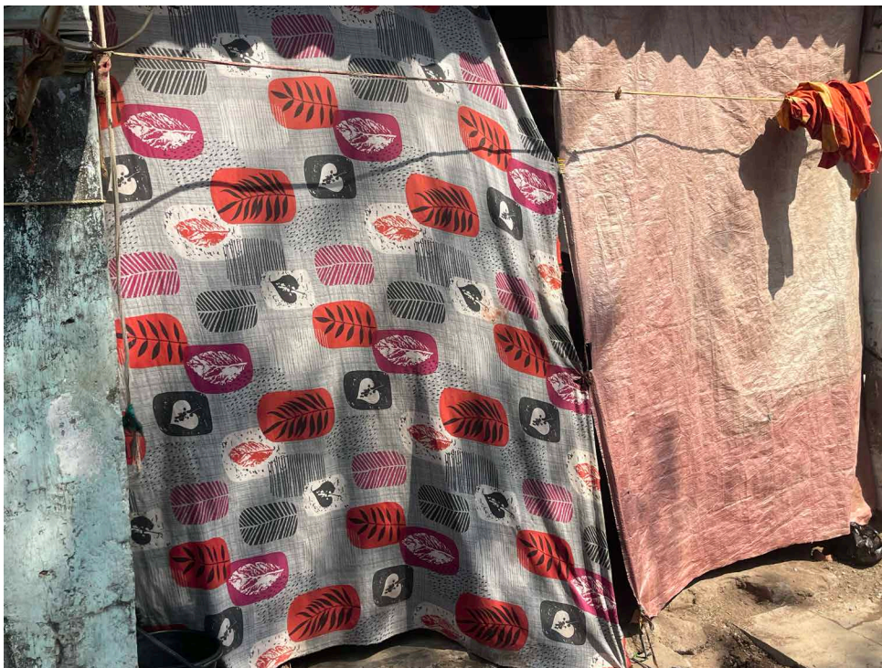
Figure 5.2.1: The image highlights the usage of full curtains covering end to end. Tied down with the help of stones, hairclips, etc. Functioning purely like a filter and deflector for air.
