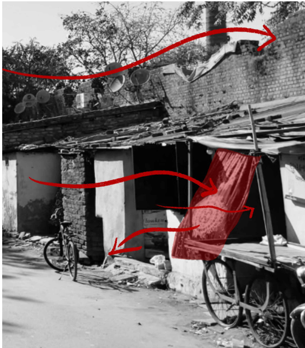
Figure 5.2.2: The image highlights the usage of curtains without any constraints. Letting it move freely as the wind comes in. It helps reduce the speed of the wind when it enters the house.
