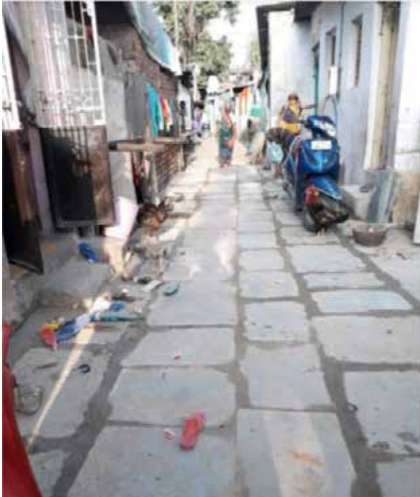
Infrastructure Improvement results in Nagori Vad, Ahmedabad
