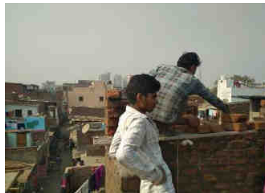
Renovation Work at a beneficiary's house
