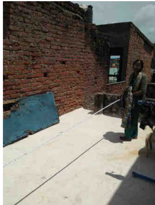
Renovation Work at a beneficiary's house
