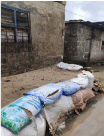
Fig 51: Sandbags wall. Source : (Nassor & Makame, 2021)
