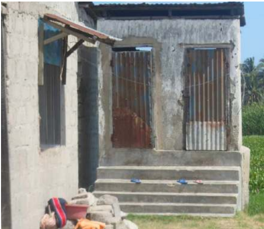
Fig 48: Pit latrine with raised foundation. Source : (Regina, 2020)
