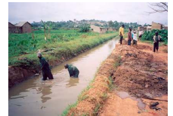
Fig 62: Removing silt from drainage channel, Kampala, Uganda Source:(Reed, 2013)
