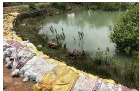
Fig 58: Flood prevention by building bunds using sandbags Source : (Das, 2020)
