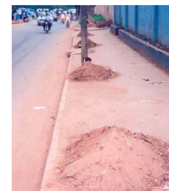
Fig 63: Silt clearance from drains Source:(Reed, 2013)
